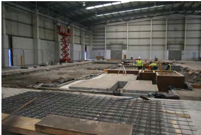
Less Common Metals: New facility being constructed
