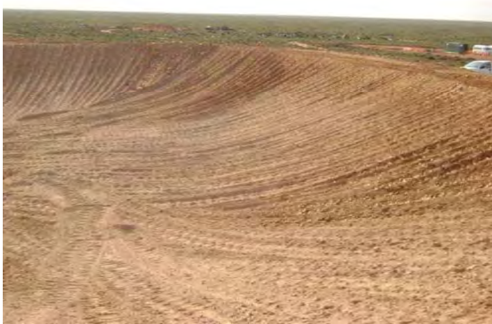
Containment pond under construction October 2011
