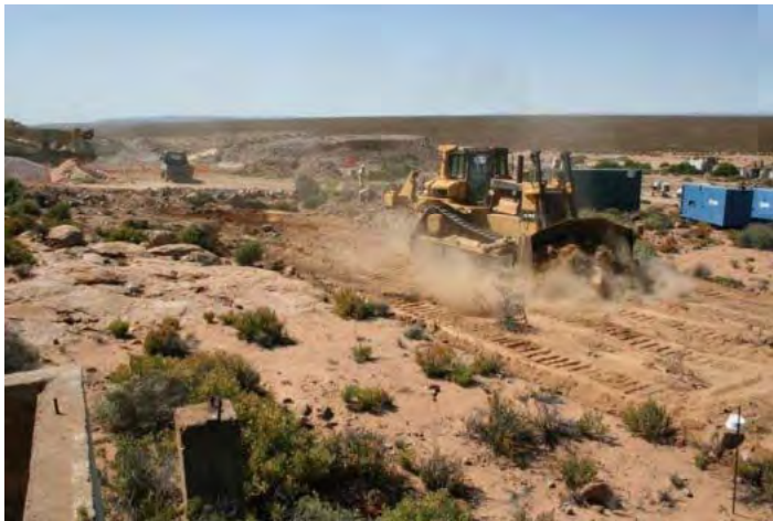
Ground prepared for buildings on outcrop bank October 2011
