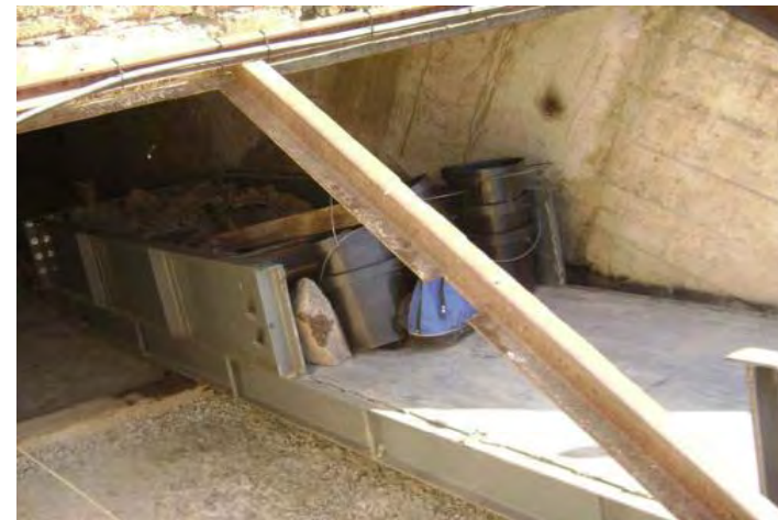
Top 45 feet of decline concrete work complete September 2011
