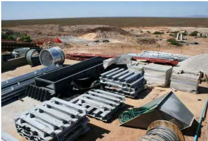
Decline refurbishment materials arrive at site September 2011
