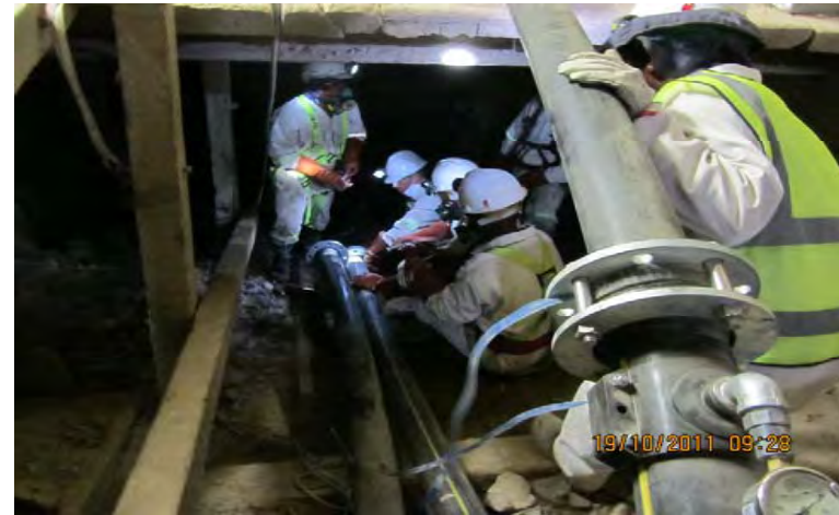
Steenkampskraal: Being refurbished for production
